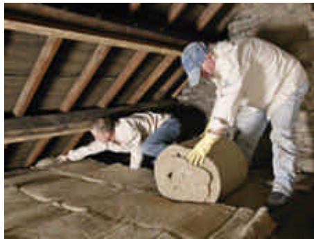
Figure 5.2 Installation of hemp insulation
