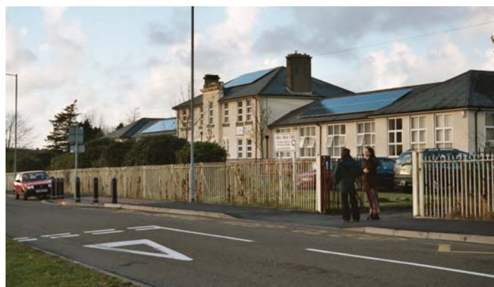
Figure 2 - Photovoltaic panels on Gwaun Cae Gurwen School.
