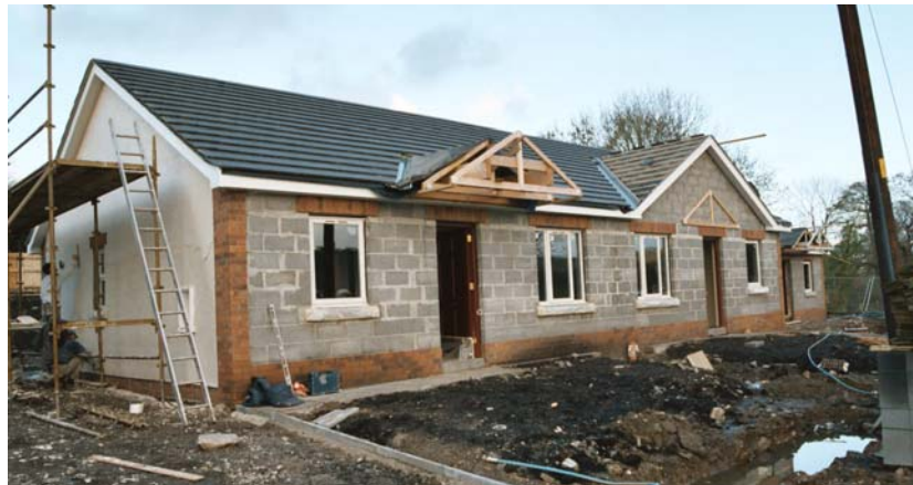
Figure 3 - Biomass housing scheme during construction
