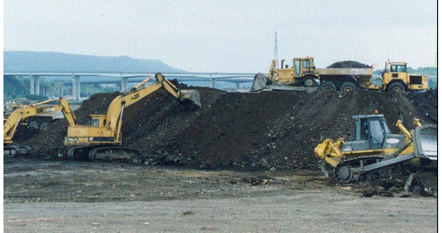
Figure 2 – Remediation works underway
