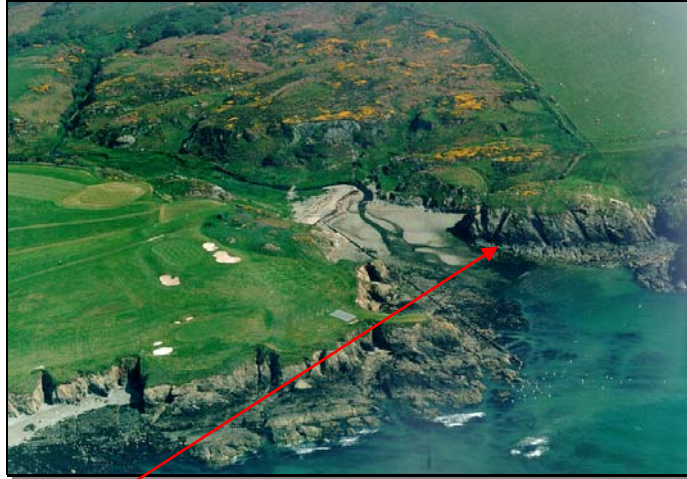
Figure 2 – Existing Aber Geirch Outfall
