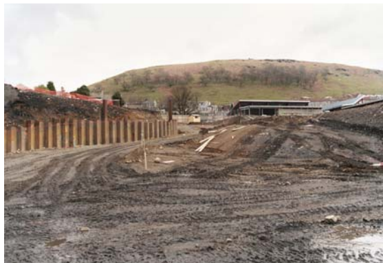
Figure 2 – Engineering works underway for modification of the road network
