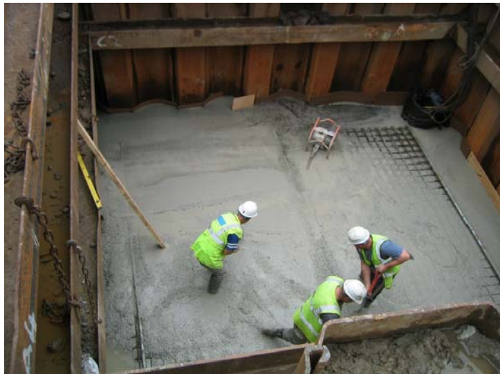
Figure 2 – Installation of replacement outfall at Gowerton.
