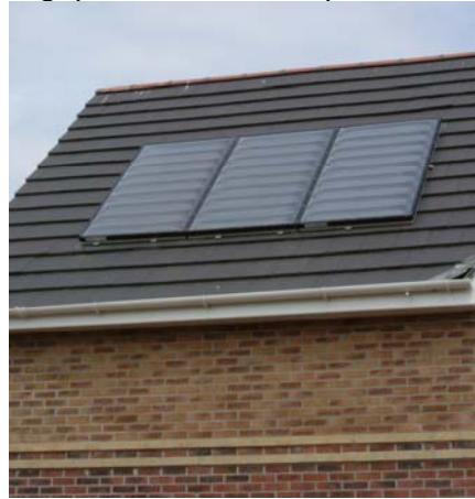
Figure 3 –Solar water heating panels on the roof of housing
