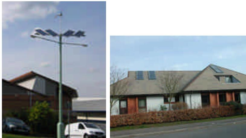
***Figure 5.3 Energy supply from solar panels and wind turbines for street lighting in car park and photovoltaic panels on a doctors surgery***
